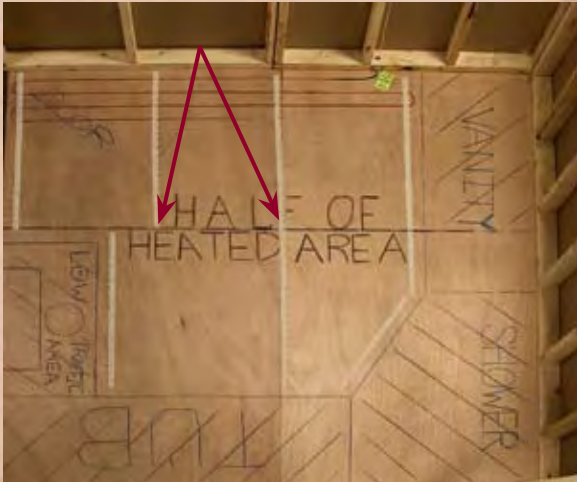
FIGURE 4a 30" distance between adjacent rows of strapping
